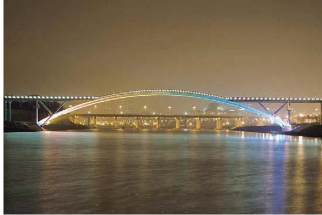
Figure (2.6): General view of Seoul footbridge
