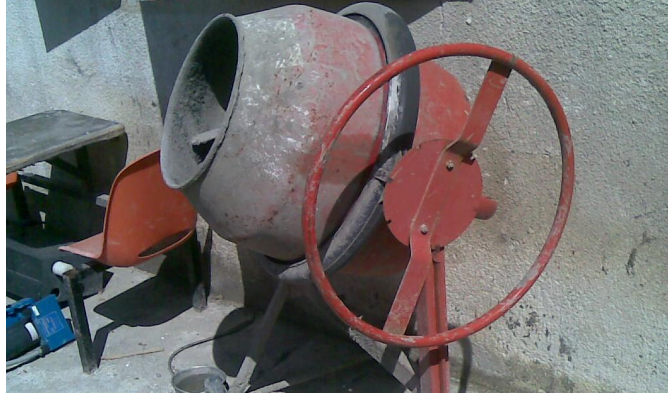
Figure (3.13): The drum mixer used for the mixing process
